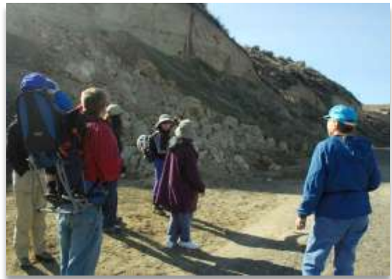
Figure 10. Recent Erosion of the Yakima Bluffs
