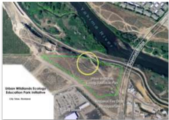
Figure 11. Terracing (Yellow Circle) to Mitigate Continued Erosion of Bluff
